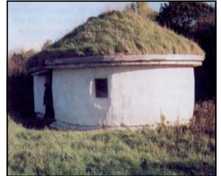
"Our house is quite simple. The inspection should take you about 10 minutes."
