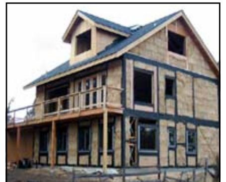
Can you huff & puff and blow this house down? (Actual photo of a house constructed of straw)
